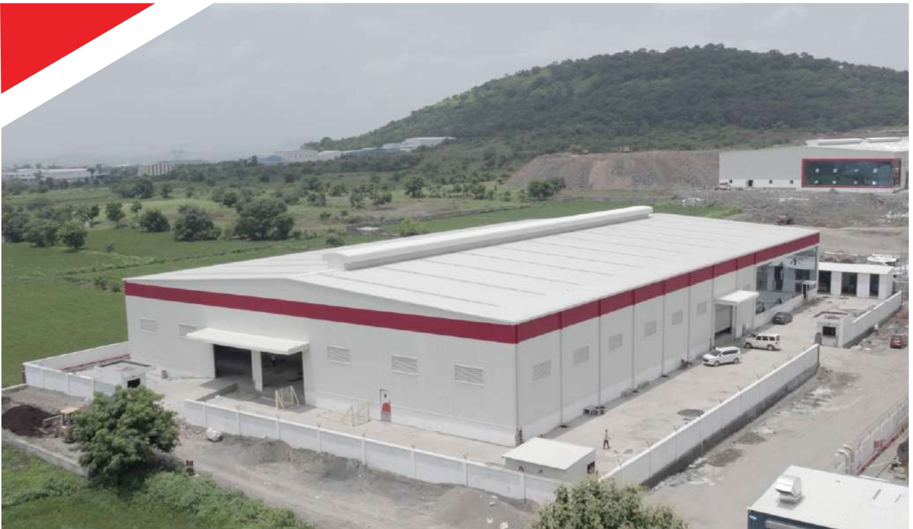
Sellowrap Industries | 3.80cr | 60,000 Sq.Ft | Chakan, Pune
